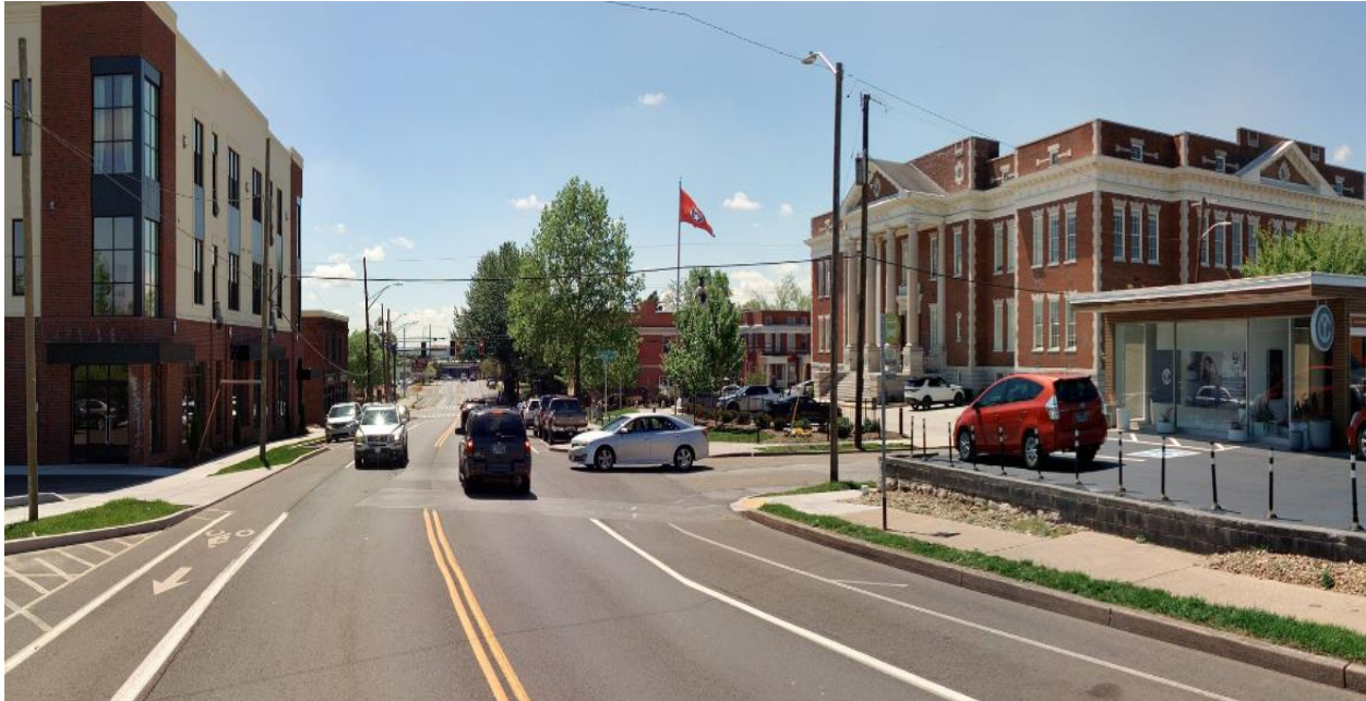
Figure 3-10 E Fifth Avenue (SR 06025), Knoxville—Suburban Context
