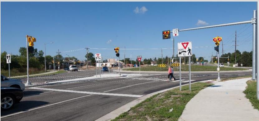
Figure 4-30 Roundabout PHB in Oakland County, MI (Suburban Context)
