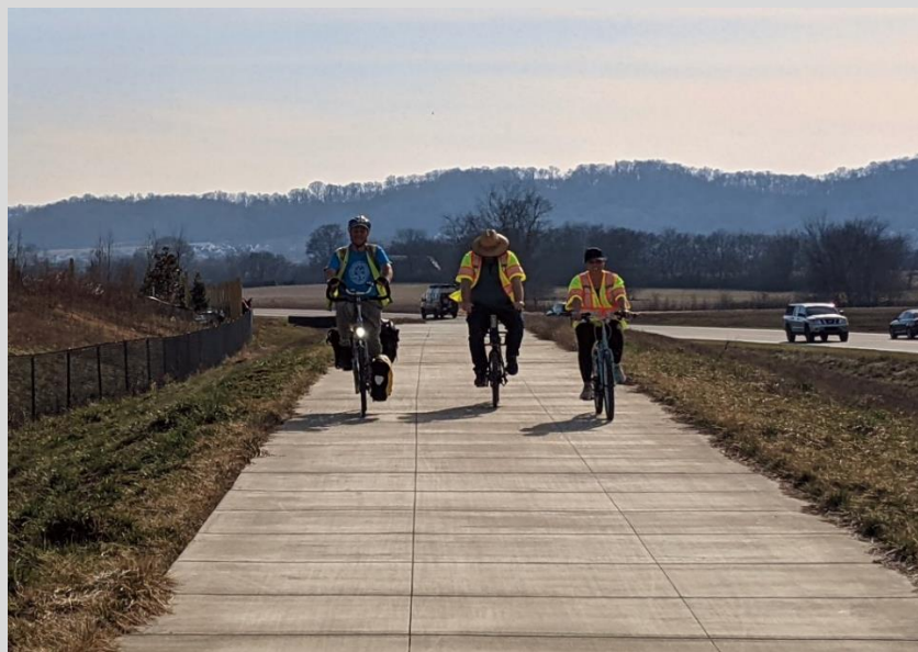
Figure 4-18 Shared-Use Path along State Route 397 in Williamson County, TN (Rural Context)
