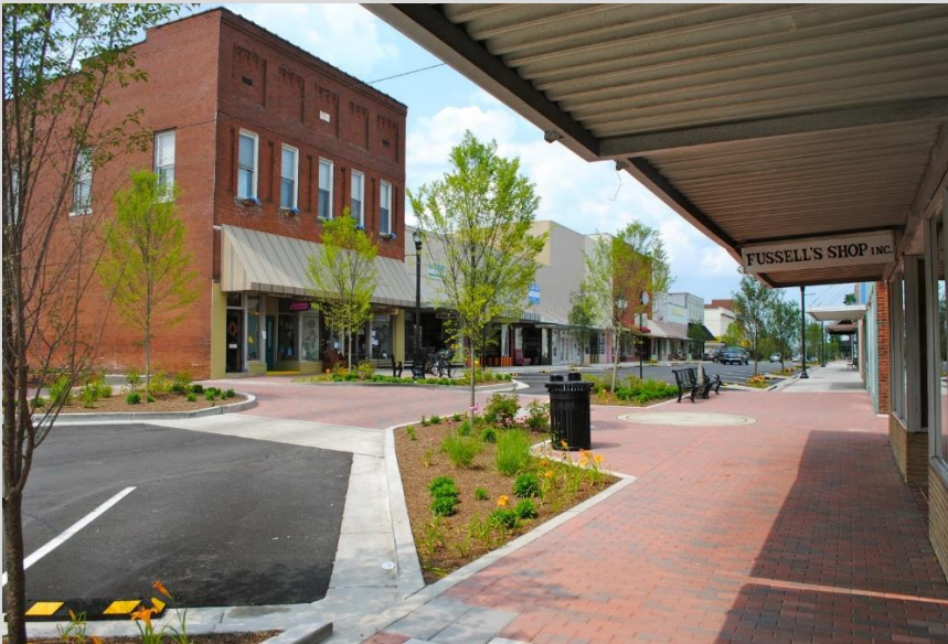
Figure 4-5 Sidewalk and Pedestrian Crossing in Dickson, TN (Urban Core Context)
