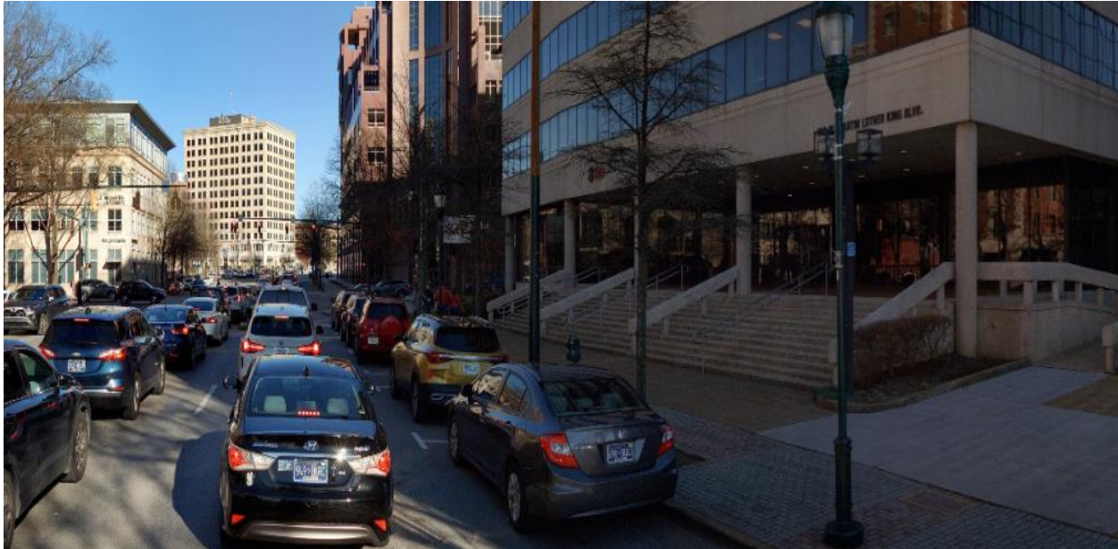
Figure 3-18 Martin Luther King Boulevard (SR 316), Chattanooga—Urban Context
