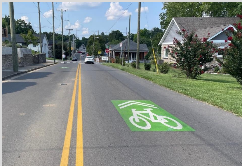
Figure 4-13 Shared Lane in Nashville, TN (Suburban Context)
