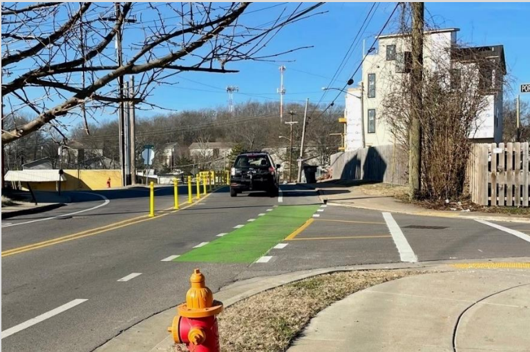
Figure 4-9 Bicycle Lane in Nashville, TN(Urban Core Context)
