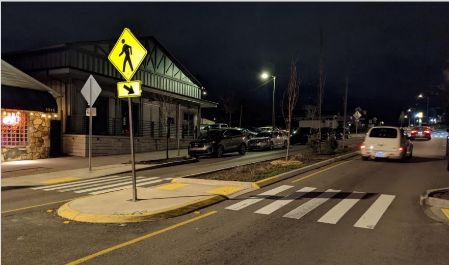
Figure 4-22 Midblock Crossing at Night in Knoxville, TN (Urban Context)
