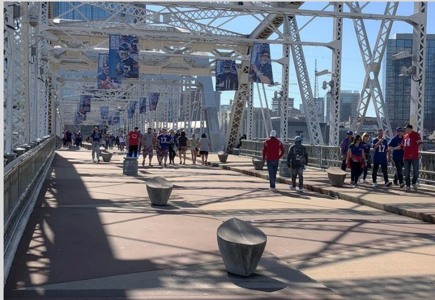
Figure 4-20 Shared-Use Path on Bridge over River in Nashville, TN (Urban Context)
