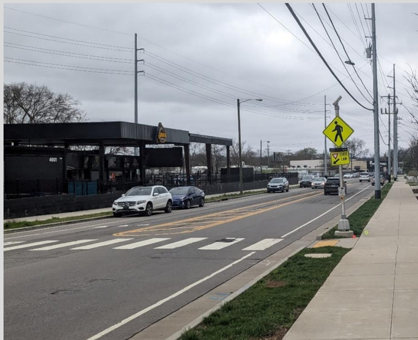
Figure 4-23 RRFB at Midblock Crosswalk in Nashville, TN
