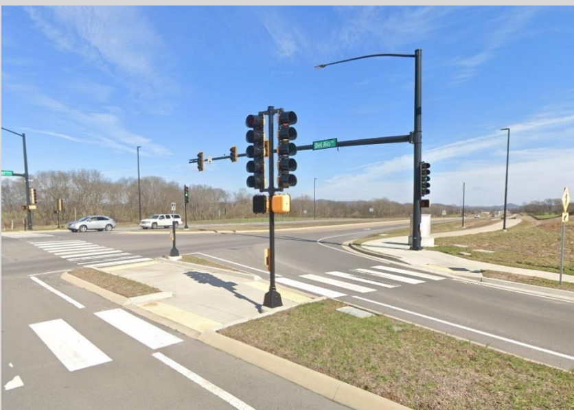
Figure 4-19 Shared-Use Path at Signalized Intersection in Franklin, TN (Suburban Context)
