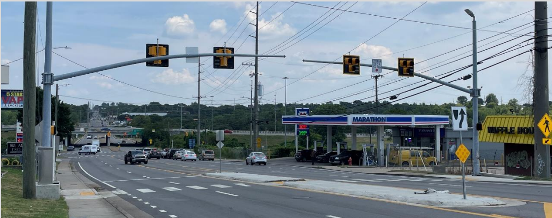
Figure 4-24 PHB at Shared-Use Path Crossing W. Trinity Lane in Nashville, TN (Urban Context)
