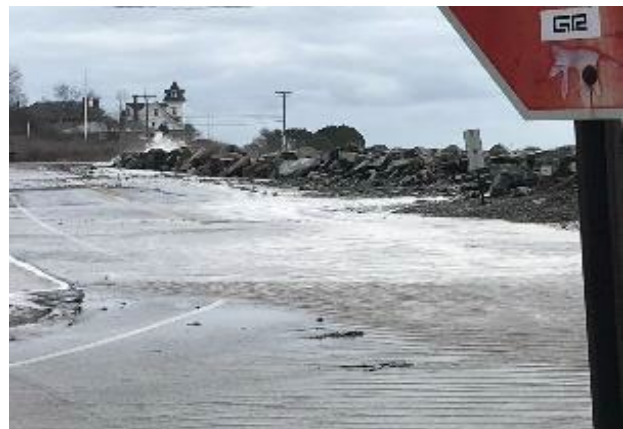
Figure 9-2. Winter Storm Riley floods Ocean Boulevard and Foss Beach in Rye, NH. Information on vulnerabilities such as this can be useful in building awareness of the need for resilience (New Hampshire Coastal Adaptation Workgroup, 2019).
