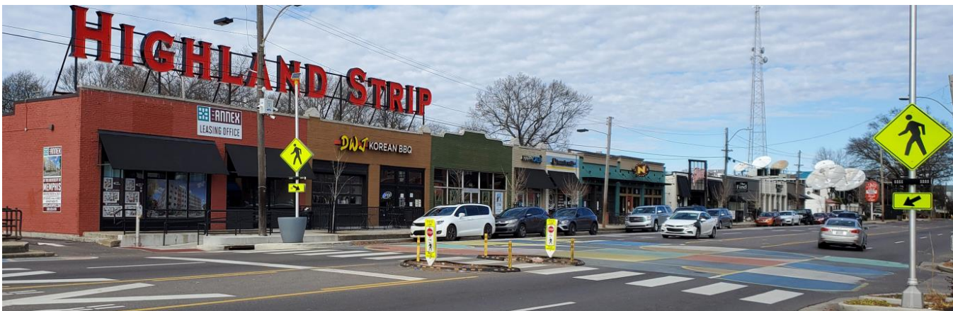
Image 2 - Memphis, TN Midblock Crossing with Continental Crosswalks, Rectangular Rapid Flashing Beacon, Pedestrian Refuge and In-Street Sign
