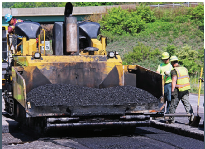
Figure 14: Using warm mix asphalt instead of standard practices produces 37 percent lower GHG emissions, according to FHWA's Infrastructure Carbon Estimator. (Photo credit: PennDOT).
