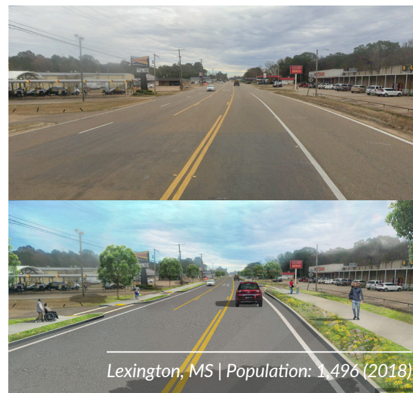
Figure 5. Example of before and after roadway conditions
