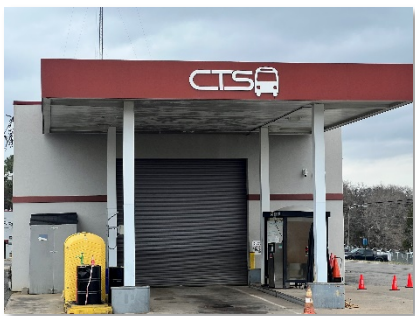
Figure 26: Bus Wash and Fueling Facility
